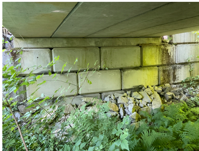
Left Bank Abutment when facing downstream
