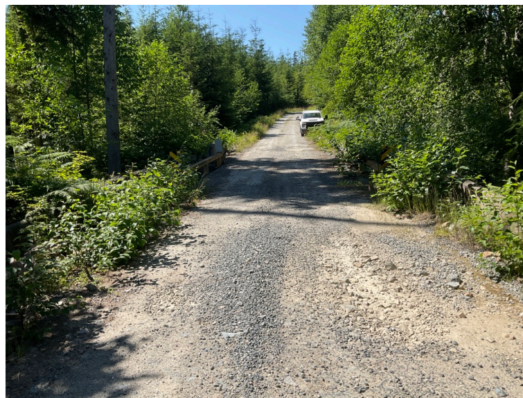
Approach from Right Bank when facing downstream
