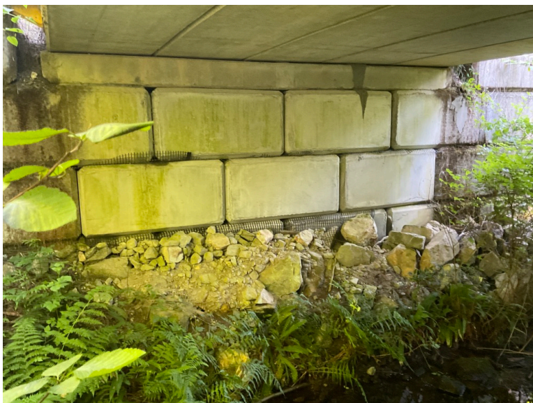
Right Bank Abutment when facing downstream
